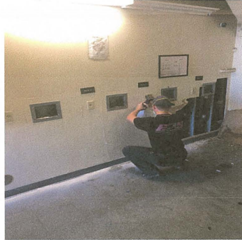
6. EPS opening 2 nd floor laundry room wall.
