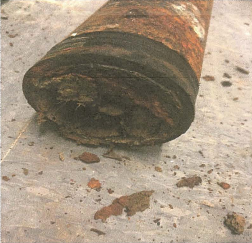
5. 1 st floor Kitchen
