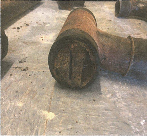
1. Inside the wall of 2 nd floor Laundry Room
