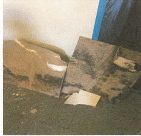
2. Inside the wall of the Laundry Room
