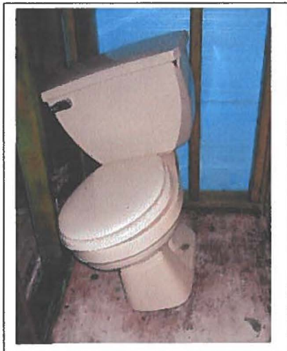
New bathroom flooring & sheetrock
