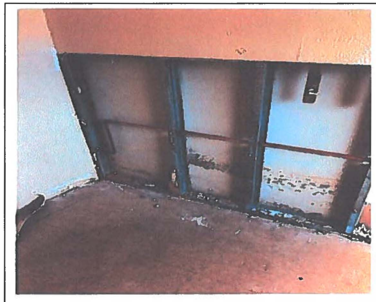
Living room area - sheetrock and flooring
