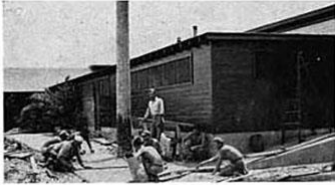
INSTALLING RAMP AND WALK, EWA
