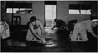
FINISHING CONCRETE
