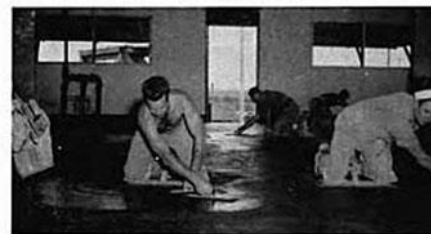
FINISHING CONCRETE SMALL ARMS MAGAZINE, EWA
