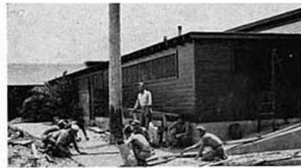
INSTALLING RAMP AND WALK, EWA
