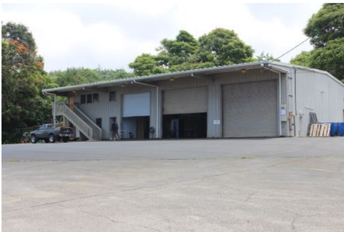
Honalō Marshaling Yard
