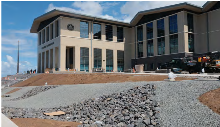
A photograph of the Kona Judiciary Complex construction site, November 2018.
