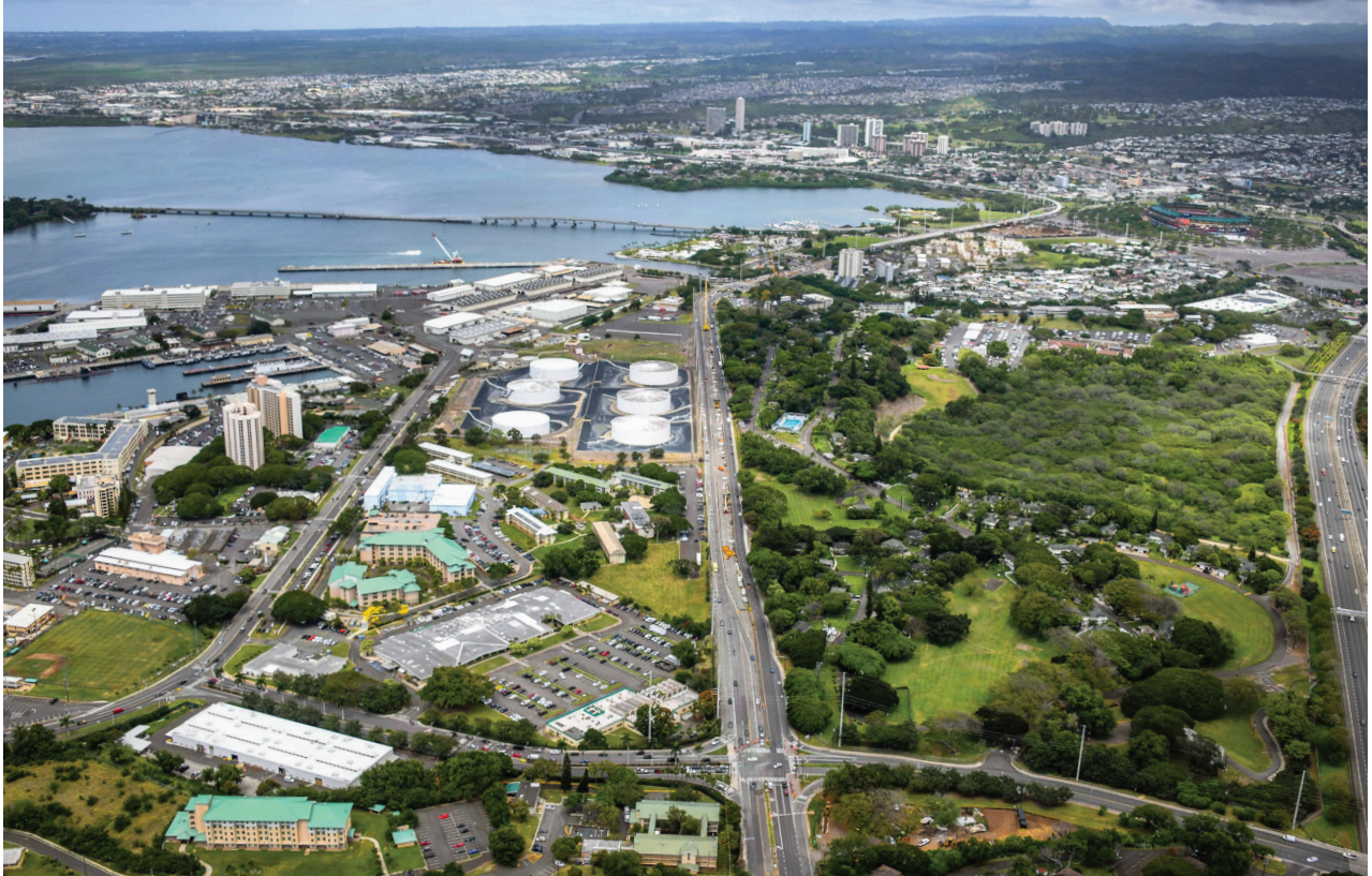
PHOTO: HONOLULU AUTHORITY FOR RAPID TRANSPORTATION
