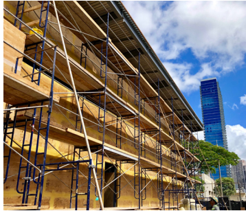
The Entrepreneurs Sandbox (Design and construction)
