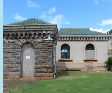
Ala Moana Pump Station Screen House and 1940 Pump Station Renovation (Design and construction)
