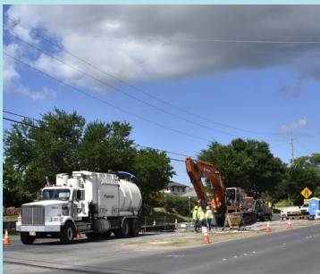
Kalaeloa Energy Corridor Phases 1 and 2 (Design and construction)
