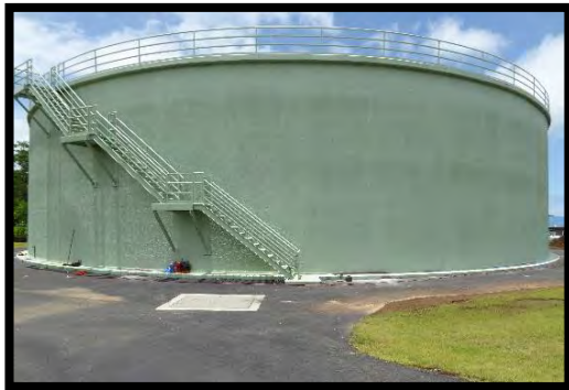
▲ New 2.0 MG tank
