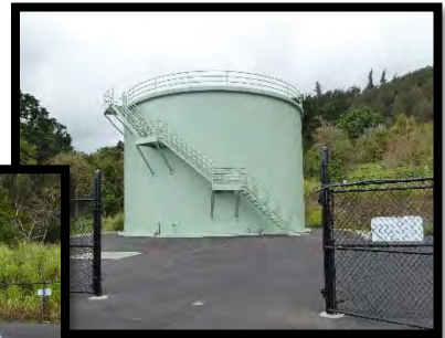
▲ New 0.3 MG tank ◀ Newly-outfitted well
