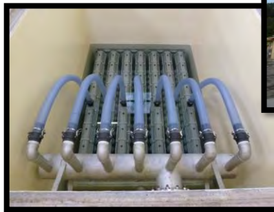
▲ New treatment building ◀ Microfiltration basin
