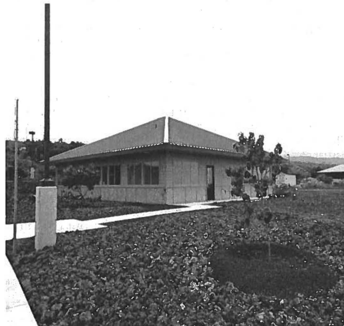
New La'i'Opua Community Center Workforce Vocational Training Center
