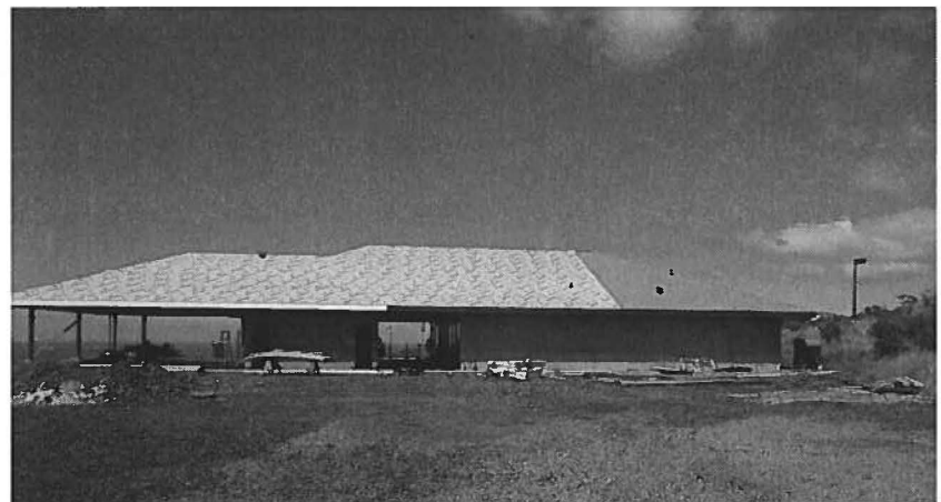
Picture of Building improvement looking North to Kohala
