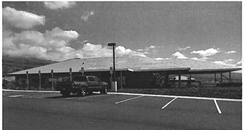
From the parking lot looking towards South Point
