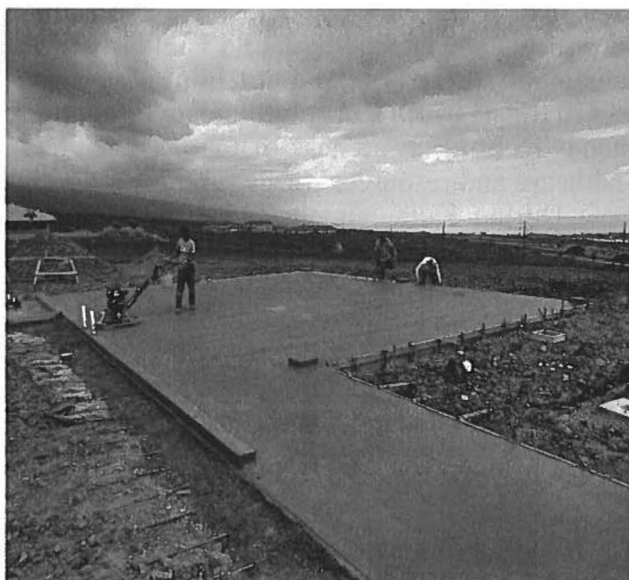
Phase 2A La'i'Opua Community Center Workforce Vocational Training Center
