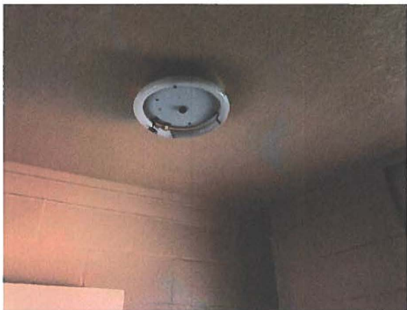
Replace Overhead Lighting
