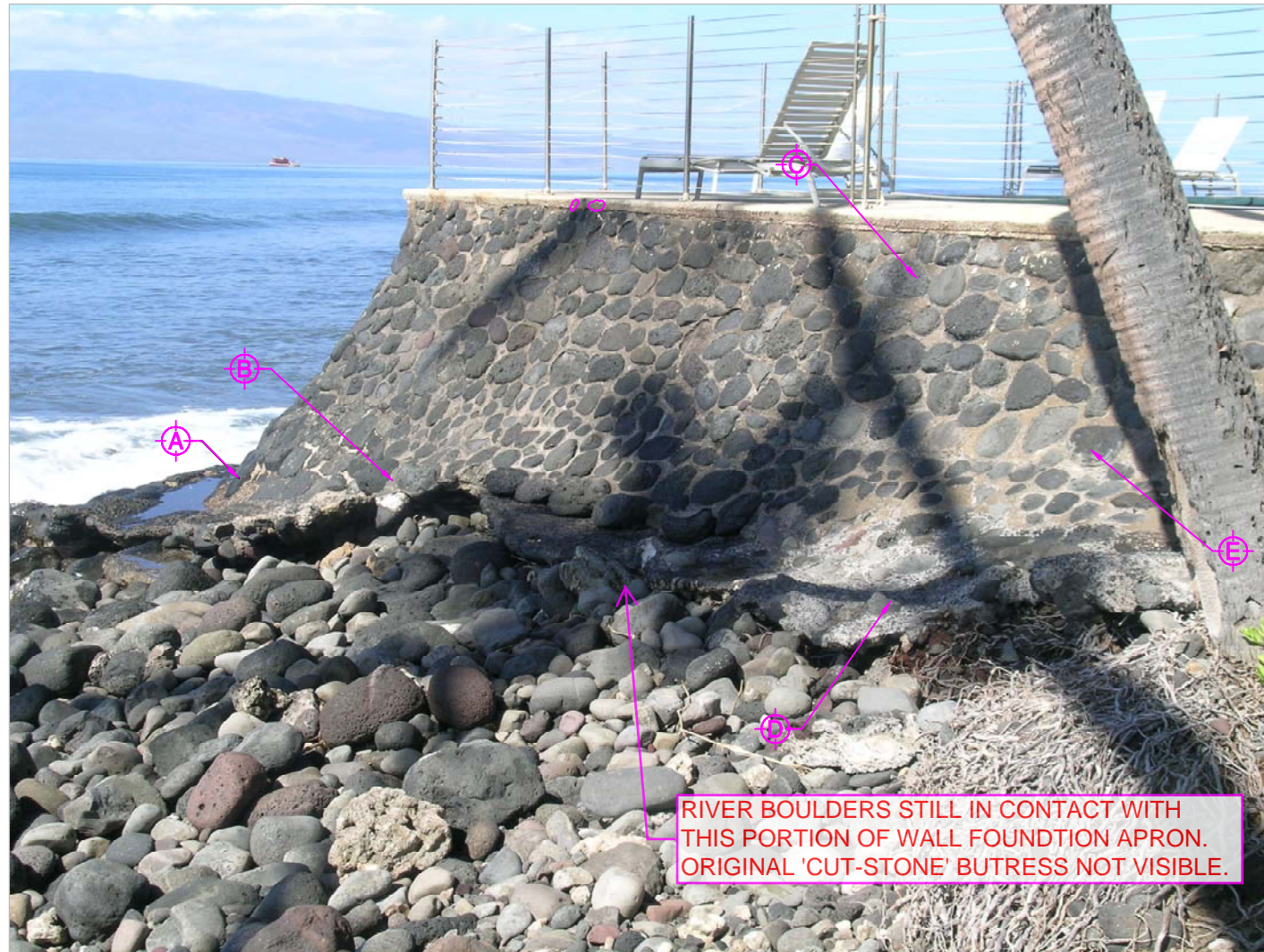
POOL WALL & FOUNDATION ALONG KA'AULA STREAM (2008)
