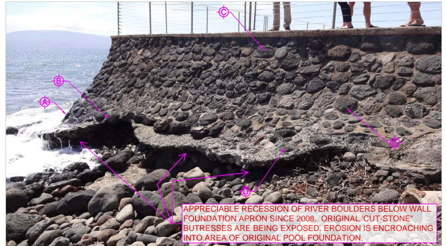
POOL WALL & FOUNDATION ALONG KA'AULA STREAM (2015)
