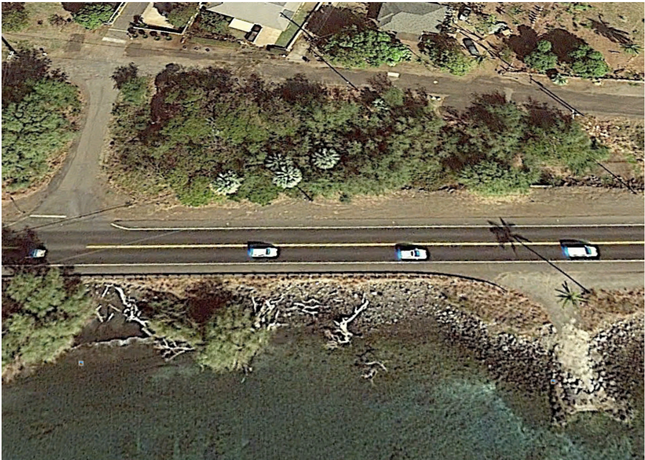
On the left side of this photo near Milemarker 14 of Honoapiilani Highway, erosion has already undermined the pavement by several feet, almost to the travel lane. The roadway here is in danger of collapse under the weight of heavy vehicles.
