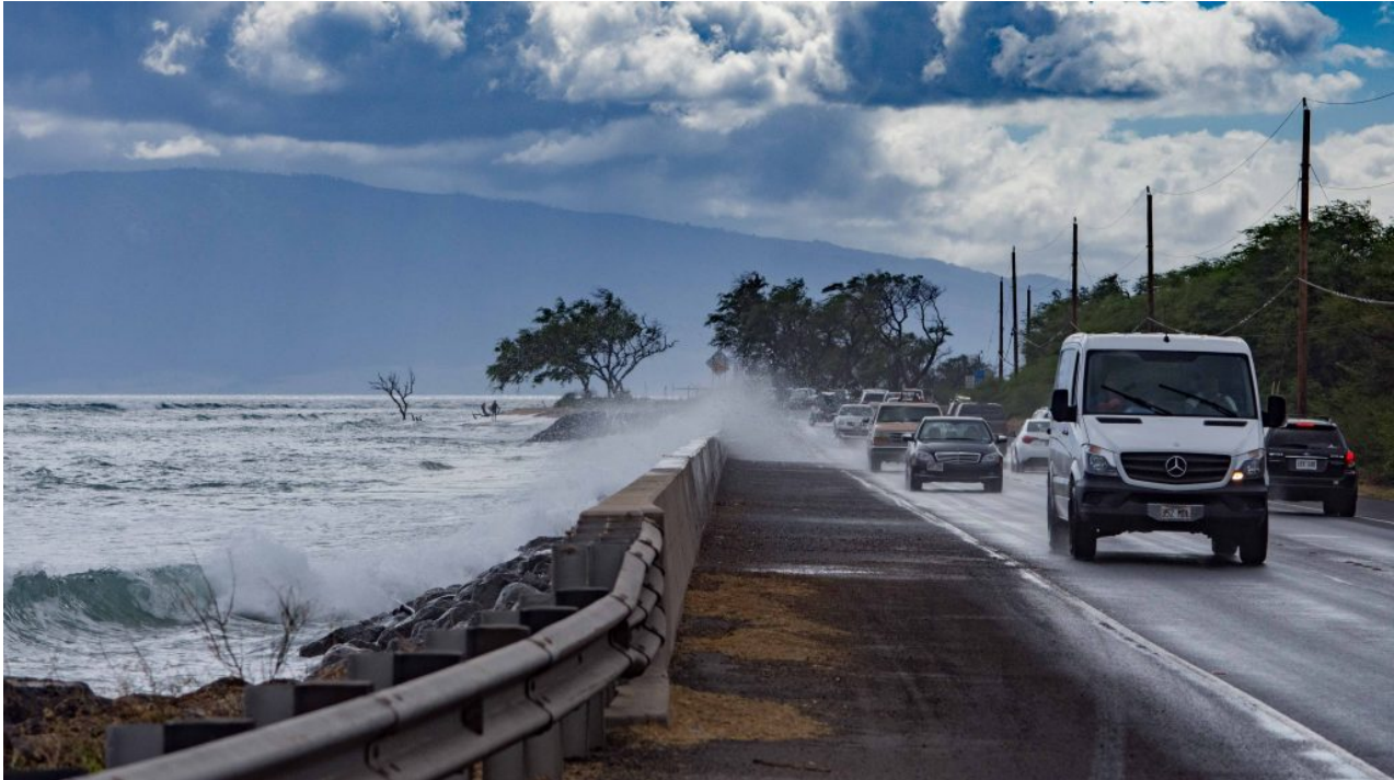
Waves overtop a seawall along Honoapiilani Highway. Vehicles are subjected to saltwater corrosion, and motorists wishing to avoid the salt water often veer into the oncoming lane, creating a serious safety hazard.
