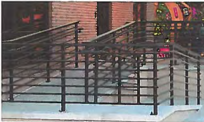
Ramp Example: Able Group Inc, Philadelphia, PA
