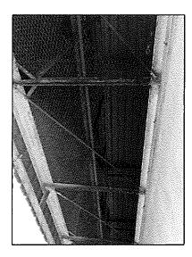
The work of replacing the grating will be done by a contractor hired by Palama Settlement. The work entails the removal of the exterior screens, cleaning and preparation of the metal so new galvanized screens may be attached, and attaching the new screens by welding. The job will require a lift, scaffolding, and hoisting and safety anchor points for workers. The contractor will be responsible for obtaining all equipment and materials.
