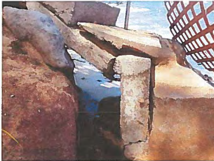
c. Two photos of erosion undercutting public beach access path, June, 2017
