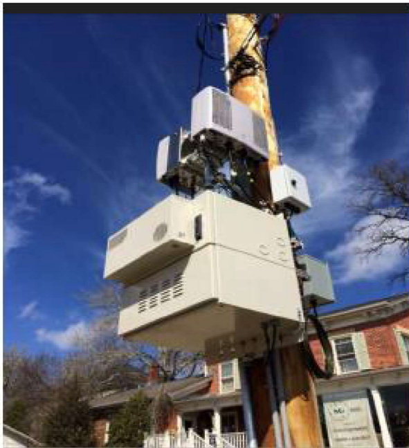
Other examples of existing Small Cell installations on utility poles.
