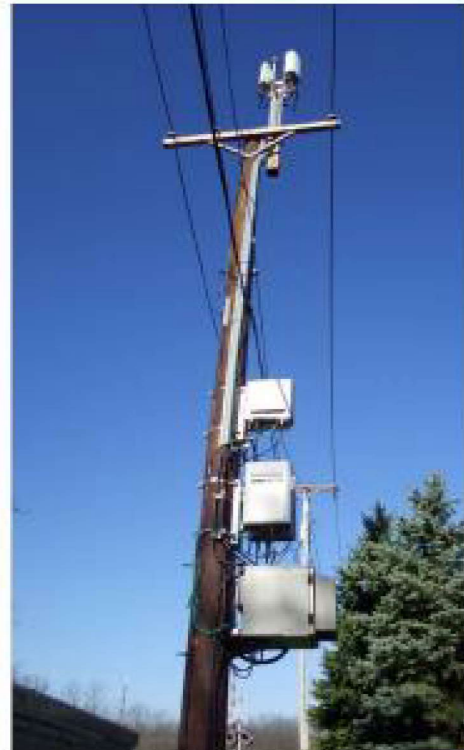
Other examples of existing Small Cell installations on utility poles.
