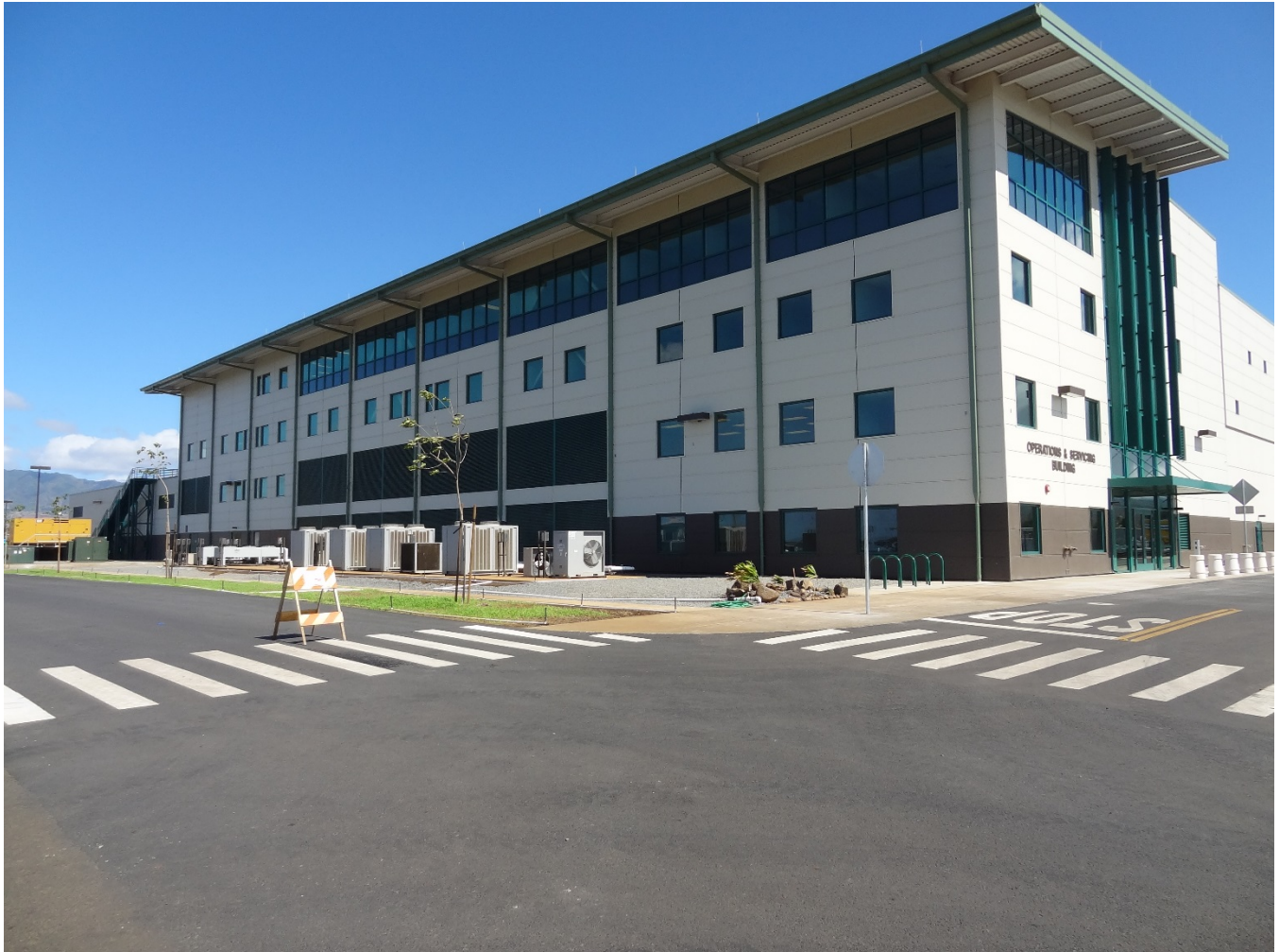
Rail Operations Center 2015
