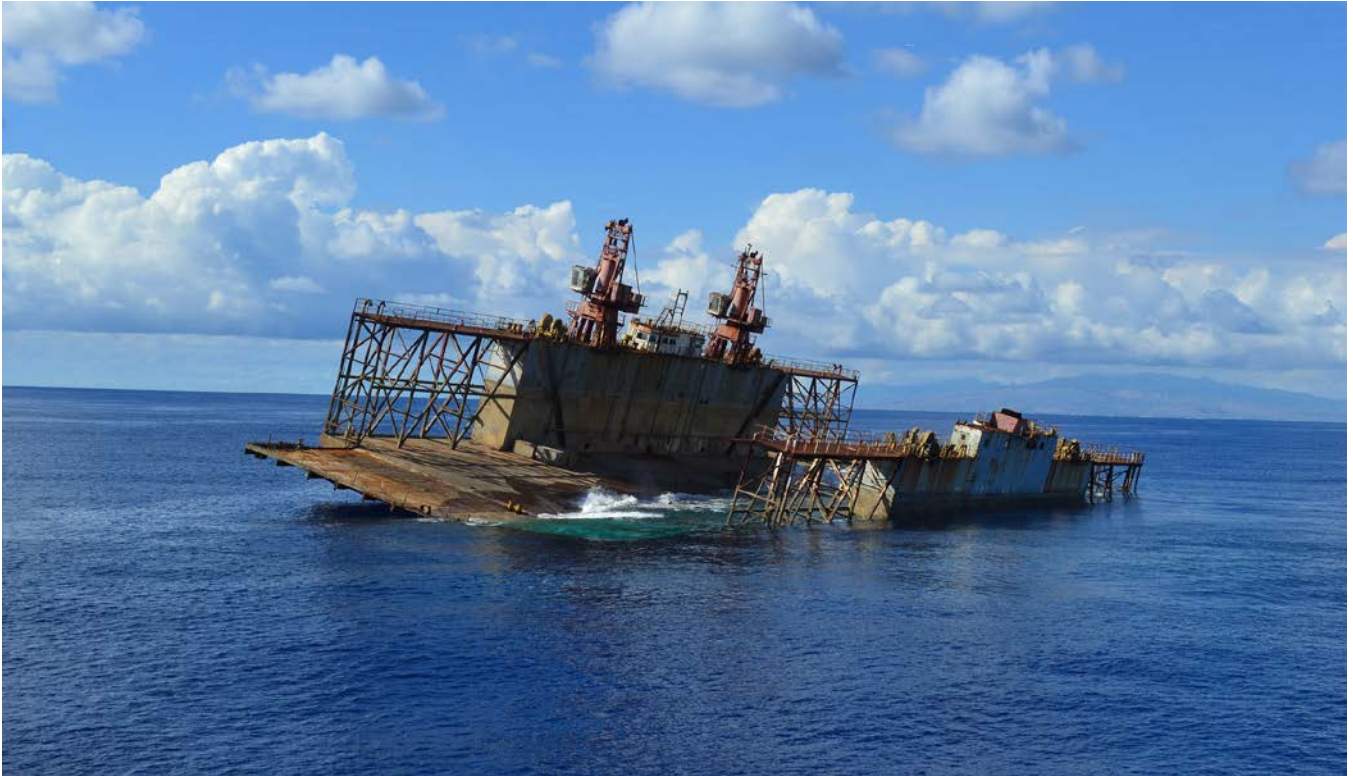
Incident Case No.: 20160203-1326 Dry Dock Disposal An abandoned floating dry dock disposed of by State DOT at sea.
