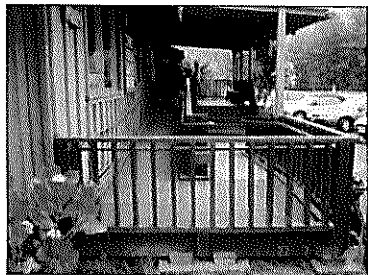
Photo: Handicap Ramp
