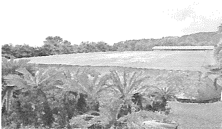
Figure 5. The 1.25 acre shade house seen from the driveway as one drives past the Royal Palms on the driveway. Here, the observer is following the road down a slight incline into the facilities site. Just over the shade house can be seen the roof of the warehouse.
