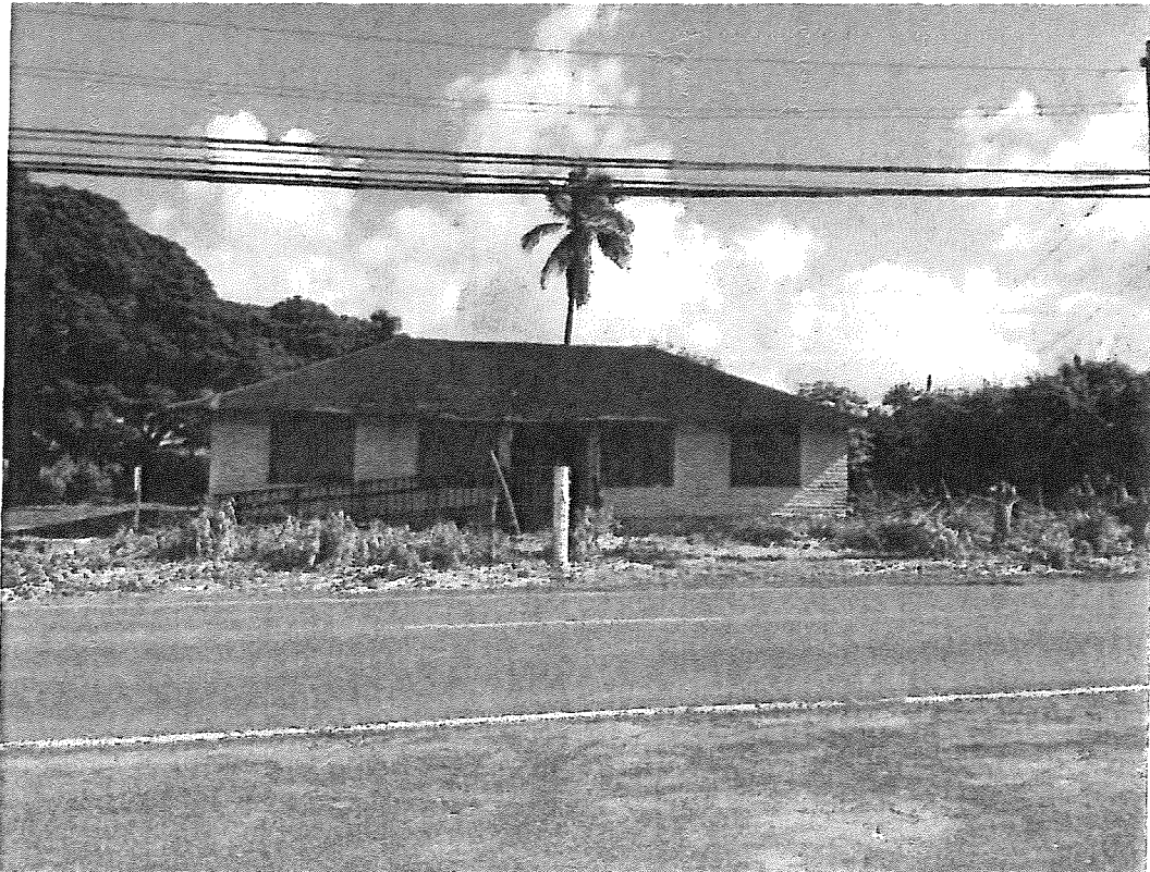
Figure 1. Existing structure and site
