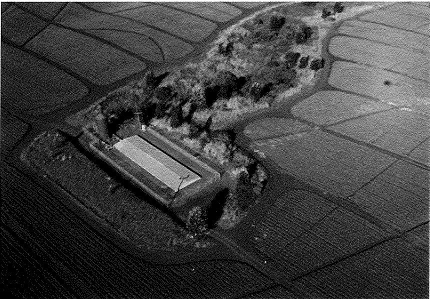
Figure 2.2-1: The below-ground potable water storage tank and aeration tower for Kunia Village. The storage tank will be replaced with above-ground steel tanks of similar capacity.
