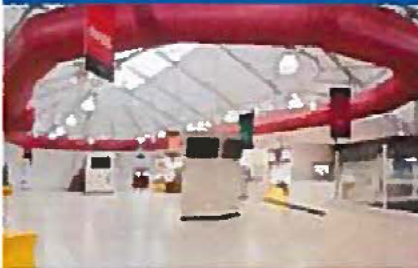
DuctSox Fabric Ducts - By Others
