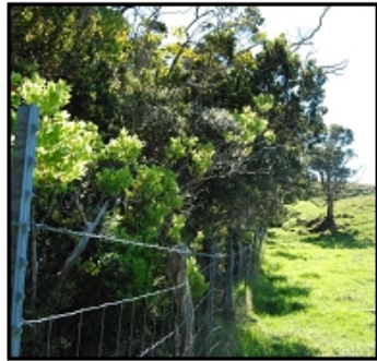
Fence construction, Puu O Umi Natural Area Reserve
