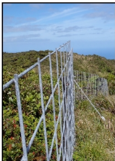
Fence construction, Kaluanui Natural Area Reserve
