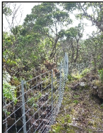
Fence construction, Alakai Wilderness Preserve
