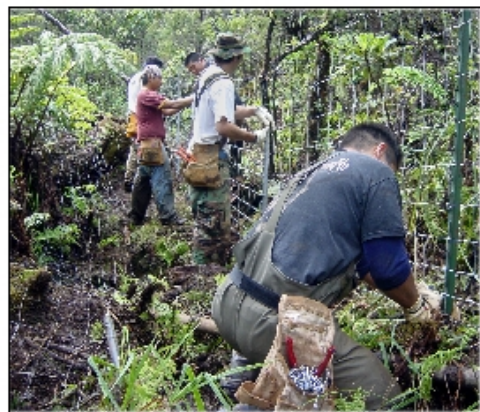
Fence construction, Hana Forest Reserve
