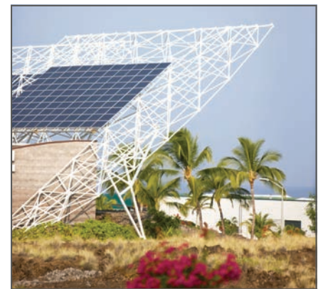
Natural Energy Laboratory of Hawaii Authority (NELHA) Gateway Energy Center
