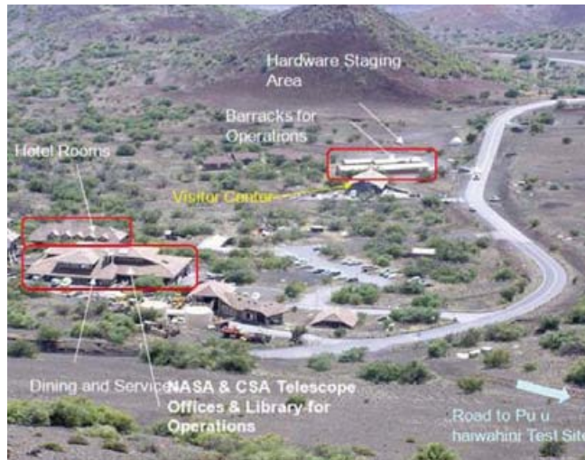
Figure 6 Hale Pohaku Facilities.
