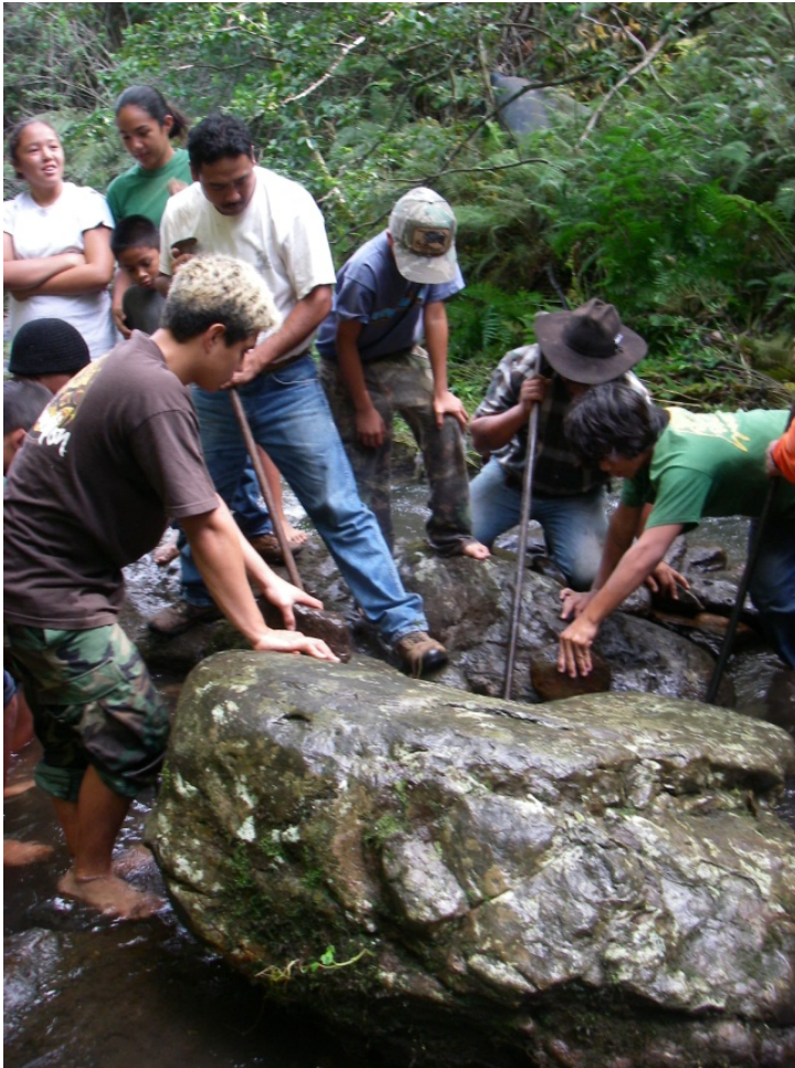
North Kohala Community members build a taro lo'i
