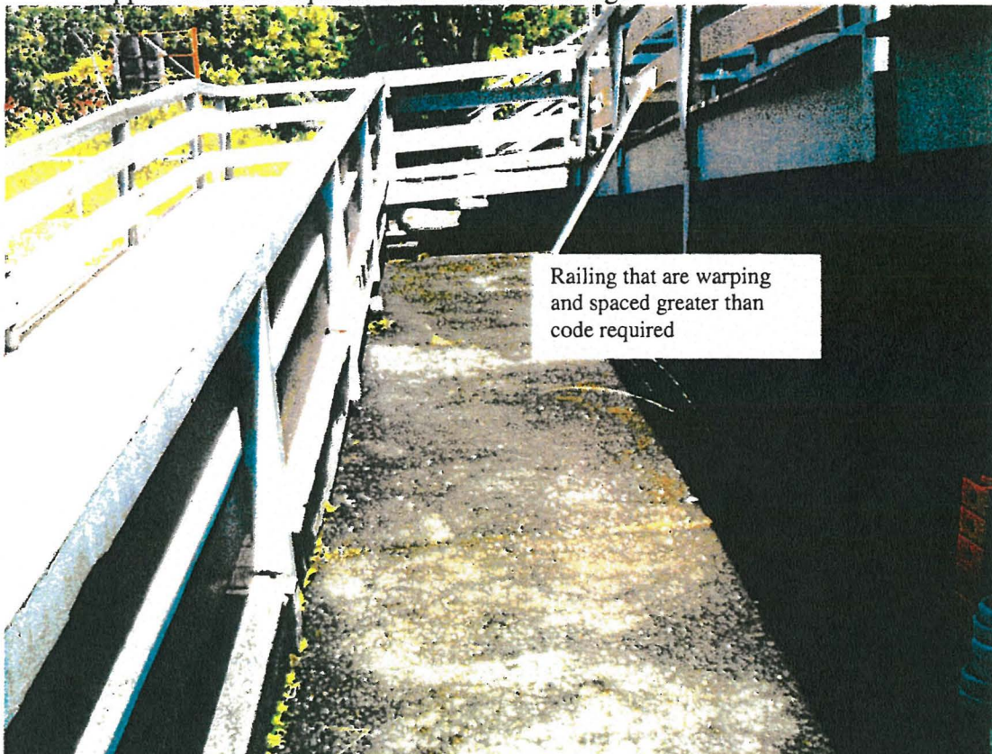
Figure 1 - West Ramp looking North
