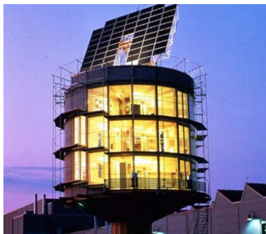
(Image via Inhabitat – home of architect Rolf Disch) The Heliotrope near Freiburg, Germany, is a rotating solar tree-house that follows the movement of the sun.
