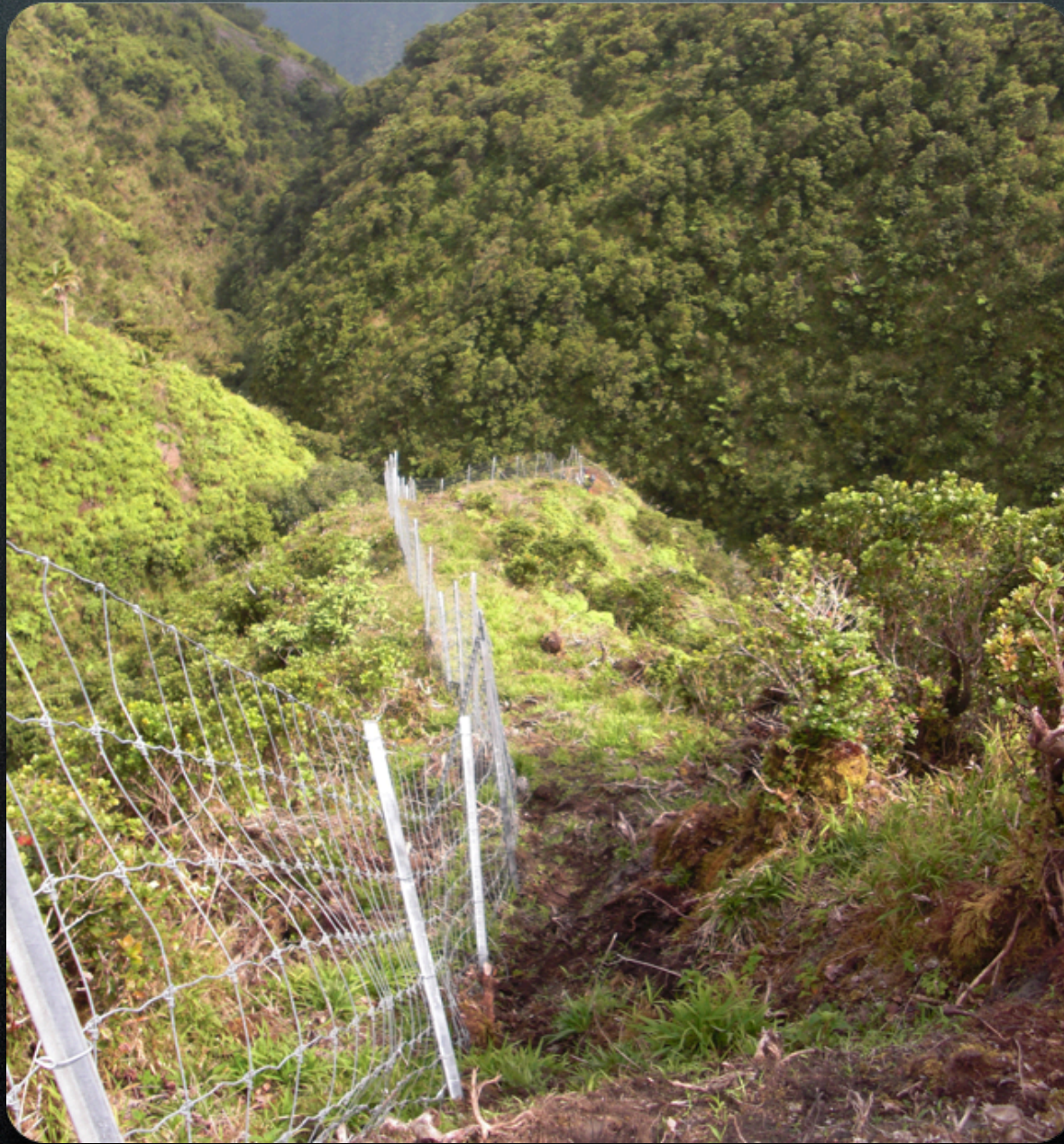
Building the fence
