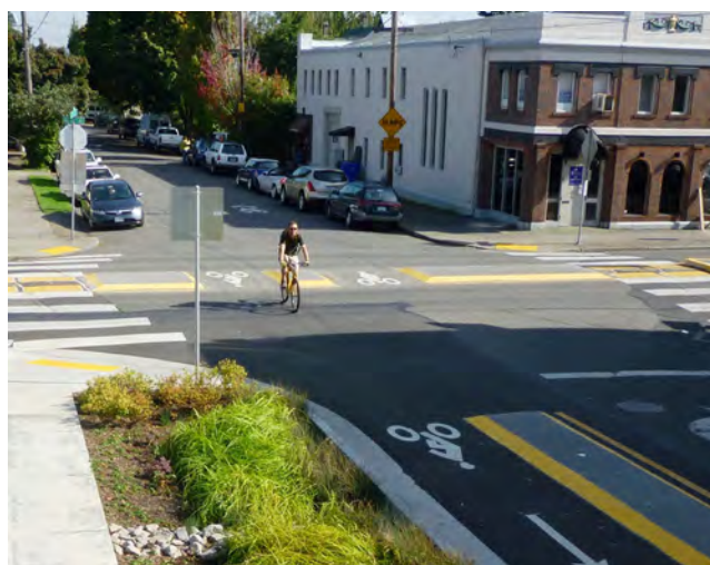
At this Portland, Oregon, intersection, bike lanes, crosswalks, and traffic lanes have been safely integrated with rain gardens that filter polluted stormwater runoff.
