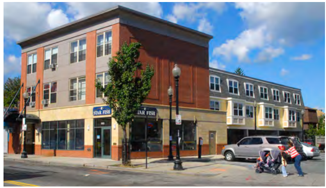
The redevelopment of Egleston Crossing in Boston's Roxbury neighborhood incorporated green building features that reduce energy consumption and utility costs while enhancing indoor air quality and improving residents' health. Photo courtesy of Egleston Crossing.
