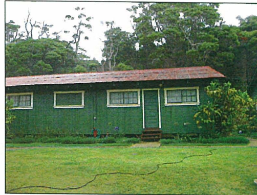
Photo: South View
