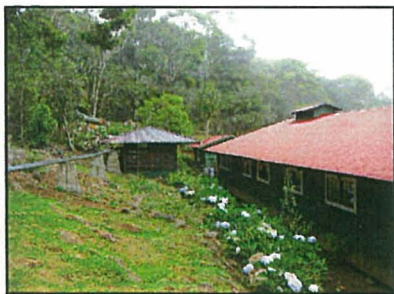
Photo: Cooler Room North of Mess Hall
