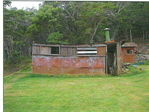
Photo: East View of Bath House
