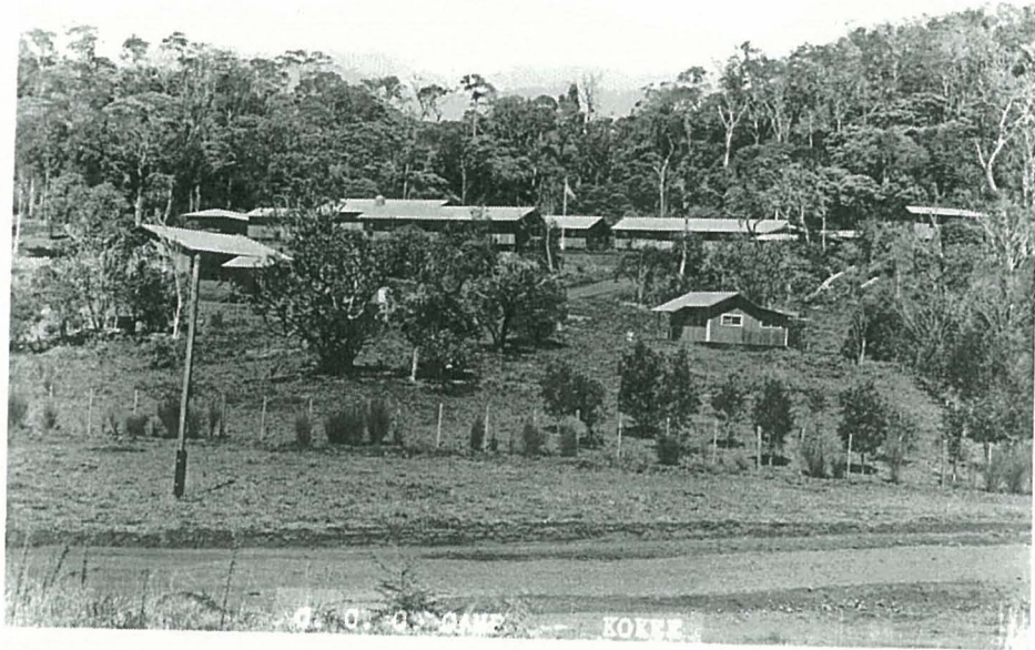
View of the CCC Camp from the South
