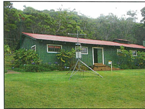
Photo: South View
