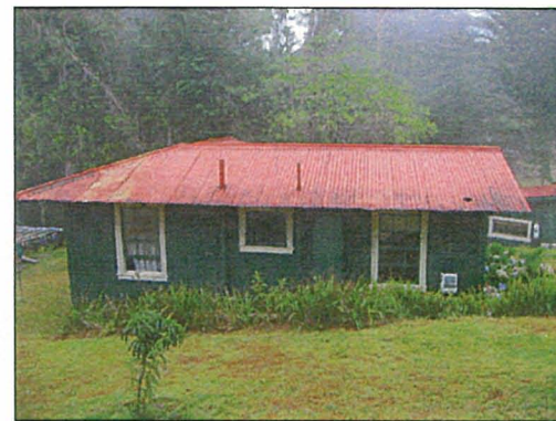
Photo: South View
