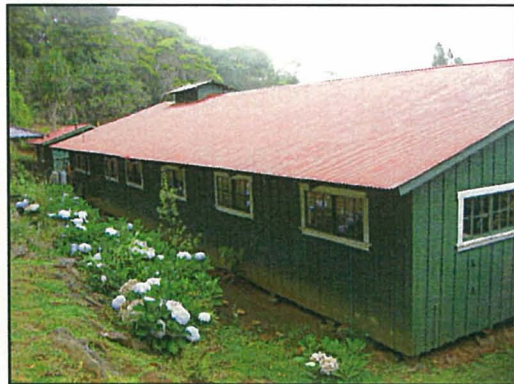
Photo: North View
