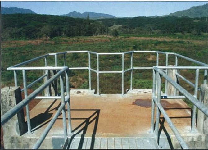
New catwalk and control gates overlooking a drained Wailua Reservoir under repair
