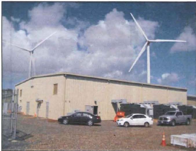
Xtreme Power BESS Building (Looking NW)
