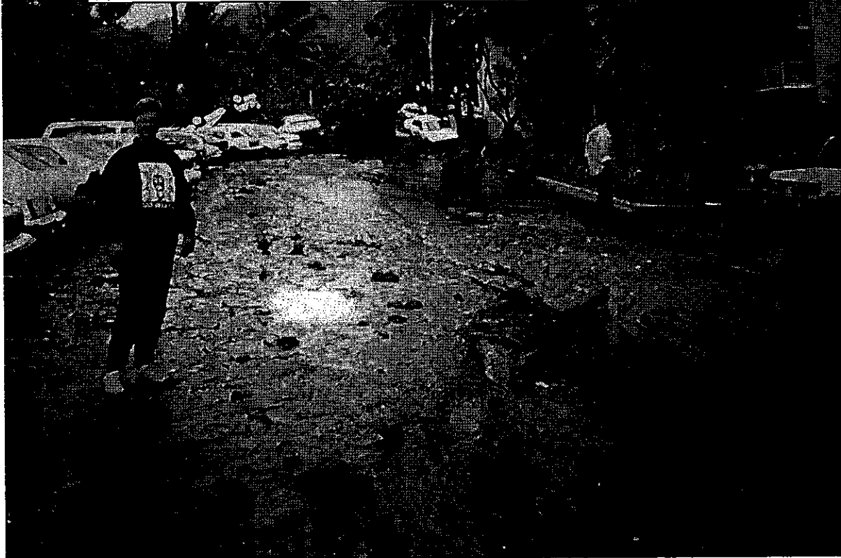
Makaha Valley Towers Parking Lot
