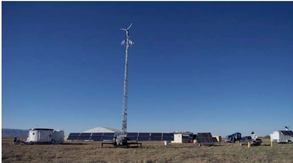
Figure 1: GSW-7000 Providing Power and Communications in Arizona Desert 2010
