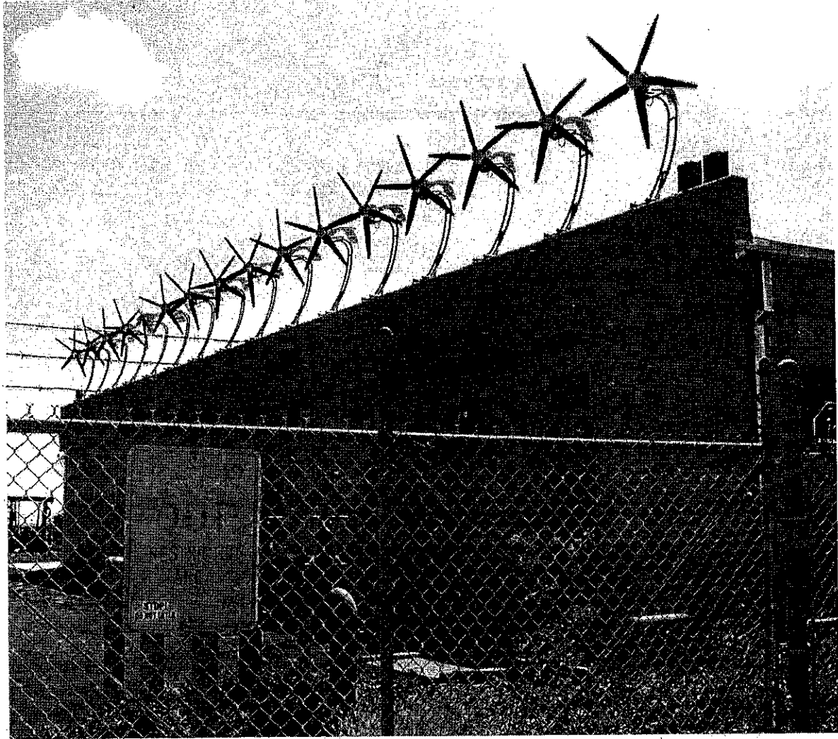
Small wind turbine array on Lagoon Drive on Honolulu International Airport property
