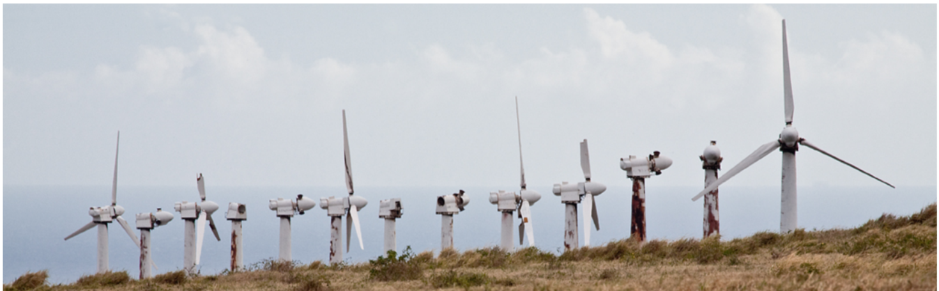
Abandoned wind power plant on the Big Island
