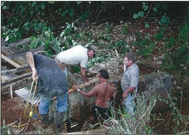
November 22 our managers and volunteers repaired a flume on Hanamaulu Ditch
