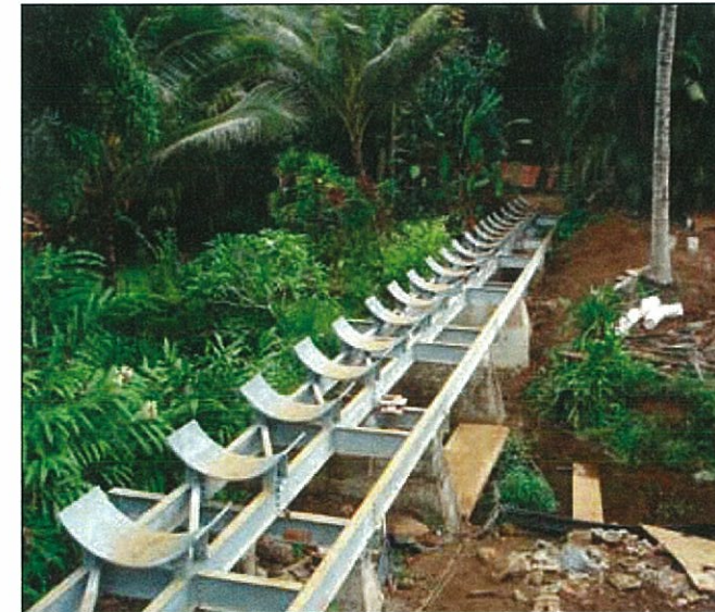
Steel supports installed for a piped replacement of a redwood flume at Kapaa stream
