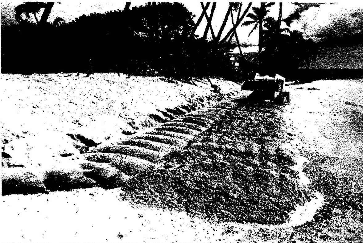
View as of 2-22-2010. Two residents have brought in tons of sand numerous times, only to have it erode. All this sand brought in will be gone after the next high tide. The sediment will travel down the beach and be deposited in the area where the beach is accreting and also off-shore, damaging the marine life.
