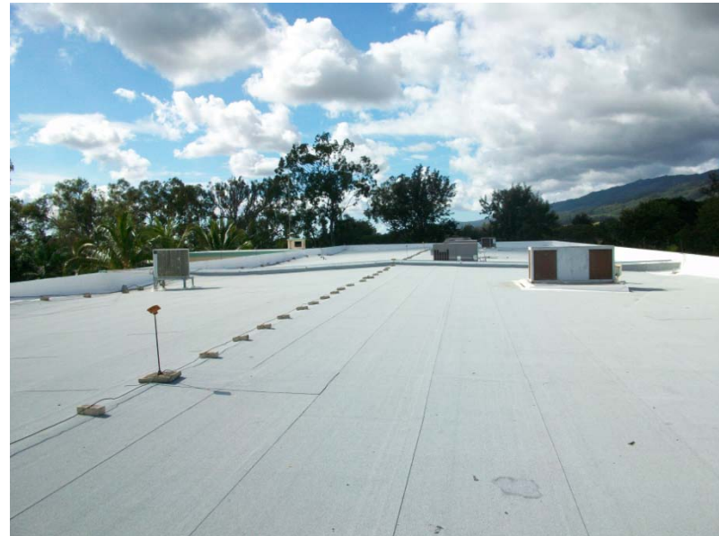
Roof with new coating
