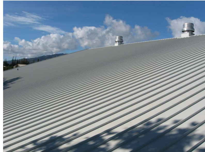
New metal standing seam roof
