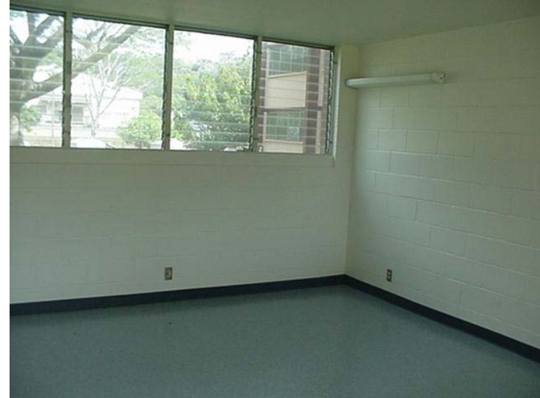
Renovated quarters at NCO Academy
