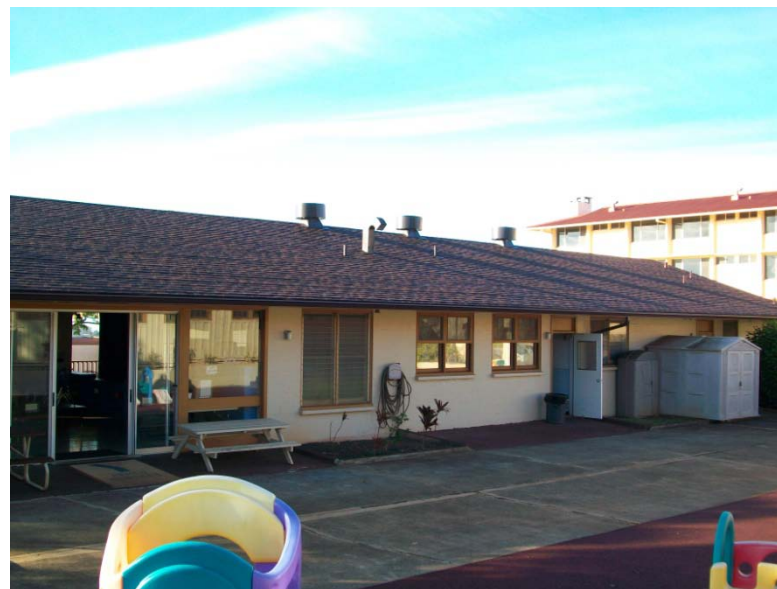
Renovated Community Facility
