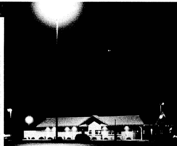
This light fixture, installed when a restaurant opened, is an example of extreme light pollution because of the amount of light it emits horizontally. People with no interest in astronomy complained about it from the first night it went into operation. Michael E. Baah
