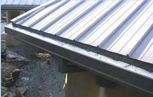
Roofing Metal Roofing
