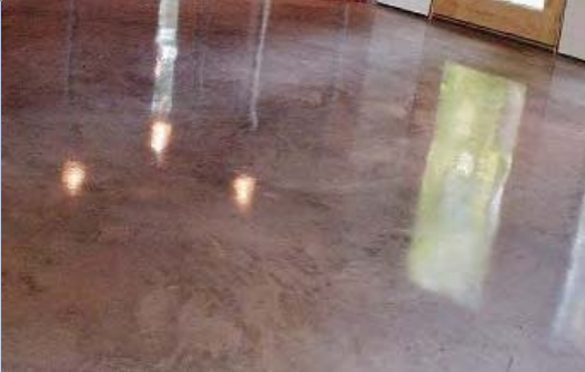
Interior Floors Glazed Sealed Concrete
