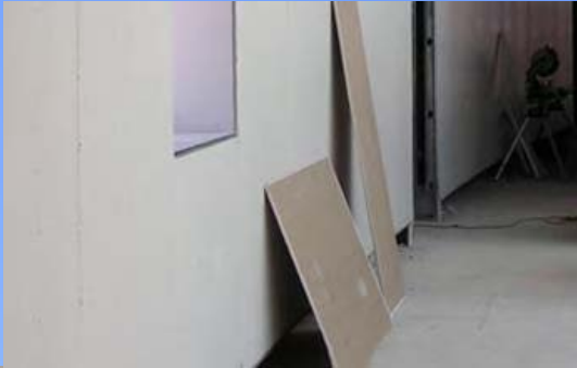
Interior Walls Gypsum board
