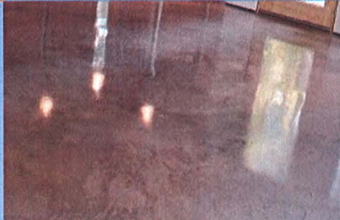
Interior Floors Glazed Sealed Concrete
