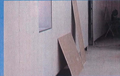
Interior Walls Gypsum board
