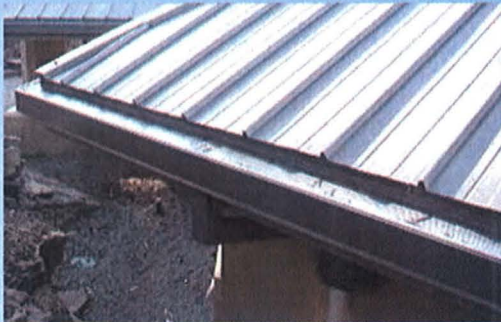
Roofing Metal Roofing
