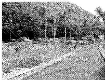
Now is a new roadway and paved parking lot
