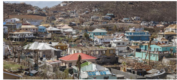
Figure 2. Homes destroyed by Hurricane Beryl in 2024.
