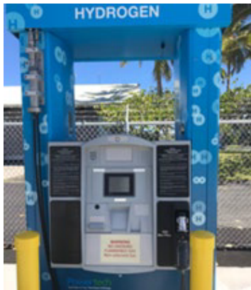
Figure 6. Hydrogen station dispenser.
