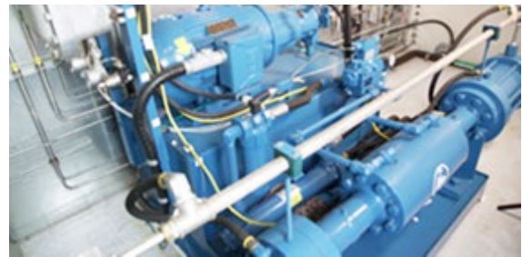
Figure 4. HydroPac compressor.
