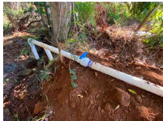
D) Newly installed end of lateral 4-inch line at drop point to South Waikapū Kuleana ‘Auwai considerably reduces water loss from Reservoir 1 nearly 1-mile upslope.
