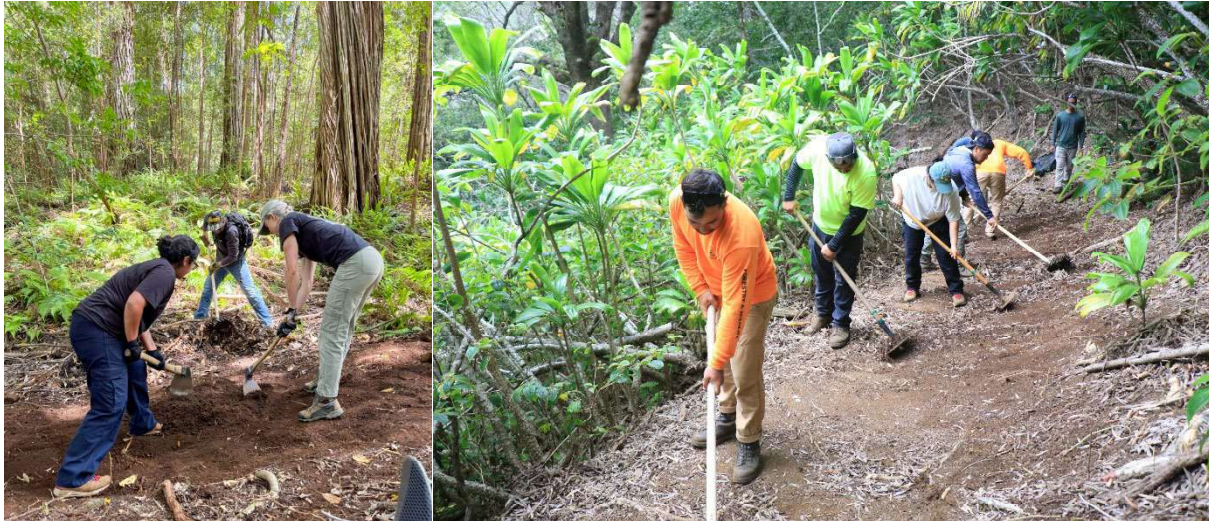
Trail crews perform maintenance and improvements to trails.
