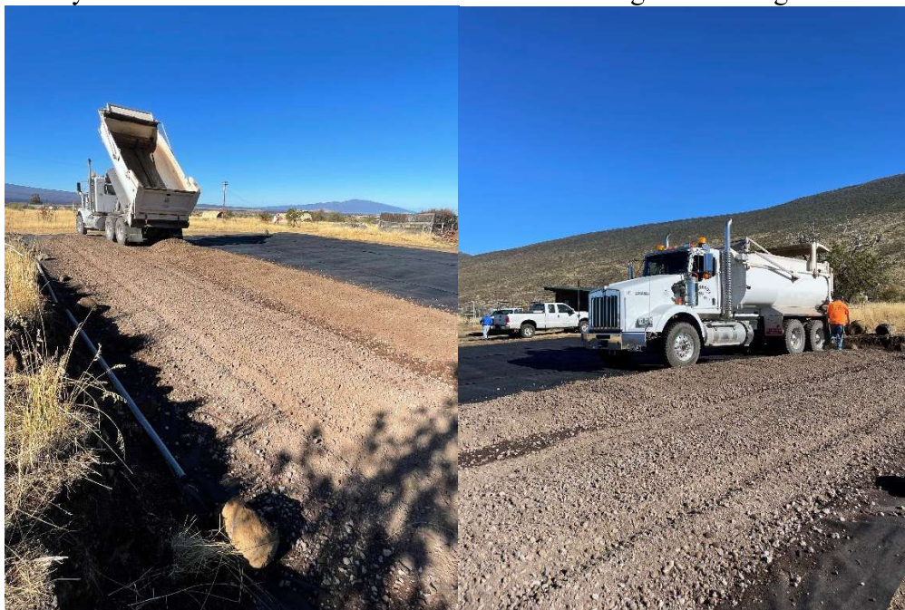
Photo 4 and 5. Delivery and spreading of aggregate material to prepare additional sites to support the East Hawaii Wildlife game program. East Hawaii
