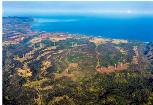
Kawailoa Wind Power, O‘ahu
