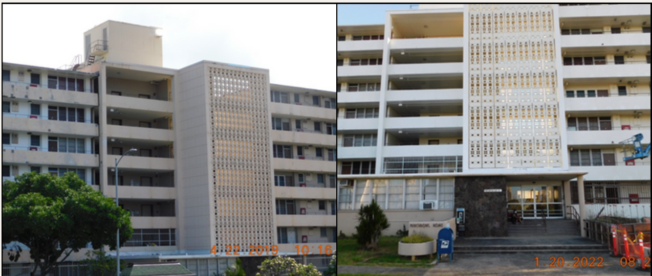
Before: Main Entry at Punchbowl Homes
