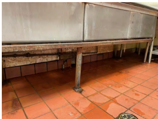
Rusted Kitchen Equipment
